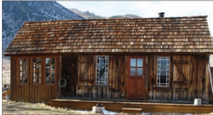
Historic cabin restored from the original built in the late 1800s.
